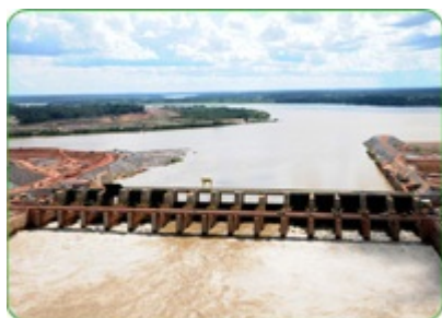
(a) Vertedouro principal
